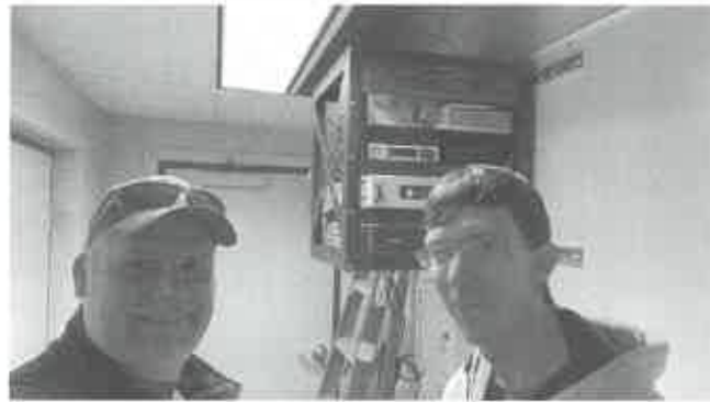
Nate and Cody ready the infrastructure in Elim
